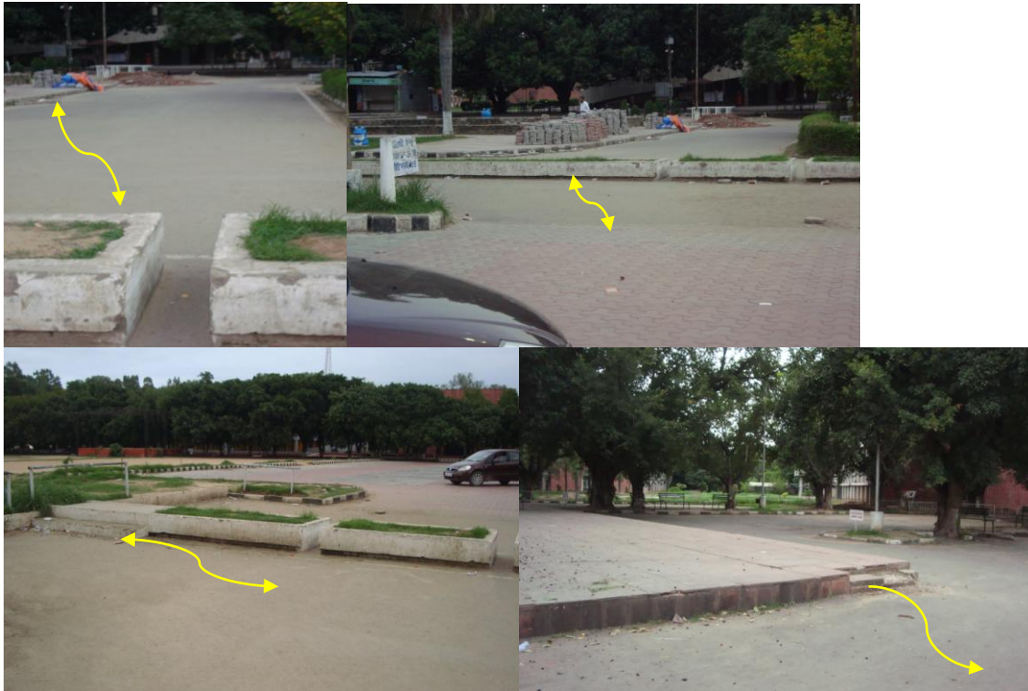
Parking Area – Cross/Jump these Cement Blocks then one can enter Student Centre
