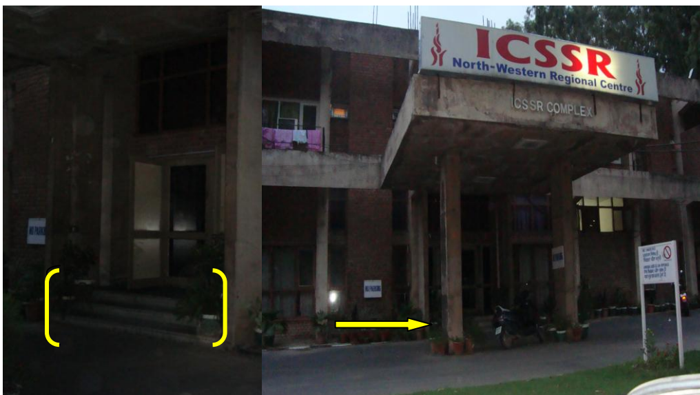
ICSSR Building - Entrance – Staircase ( Seminar Halls)
